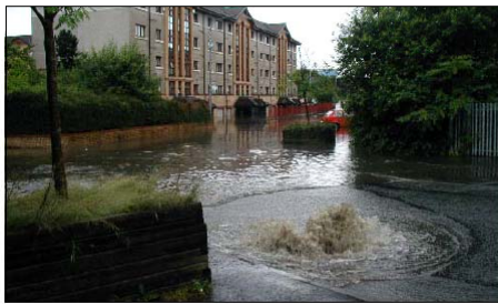
Figure 3.4 Glasgow Flooding 2002 Showing the Exceedance of Sewerage Capacity (courtesy Scottish Water)
